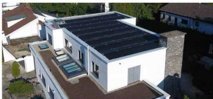
PVT system integrated into a flat roof of a detached house in Germany Photo: EVO Deutschland GmbH
