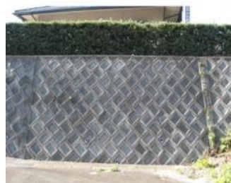
練石積み造擁壁
