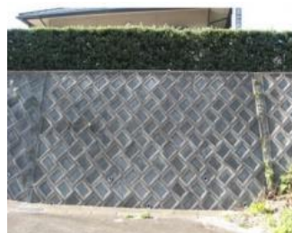
練石積み造擁壁
