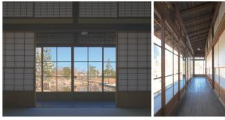
Of the Shoin's original materials, about 60% survived. Beams, roof frame, roofing tiles and other missing parts had to be replaced. Fortunately, much of the material from the interior remained, making it possible to restore it to its pre-demolition state.
